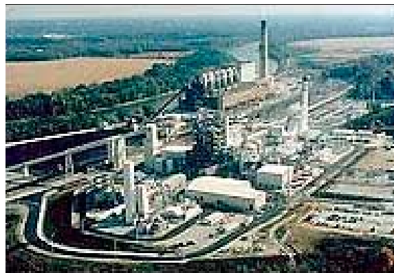
The Wabash River Clean Coal Power Plant
